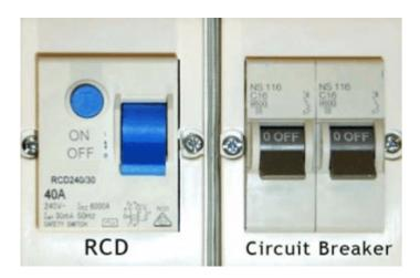
A RCD looks like a circuit breaker, but also has a test button. The photograph shows two circuit breakers compared with a RCD (note the test button). Combined RCD/circuit breakers are available also. These devices provide protection from overload, short circuit and electrocution. They also have a test button.
